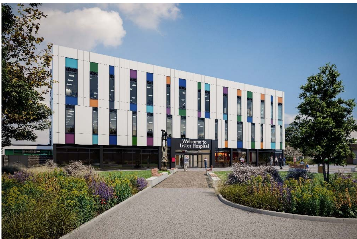
* An indicative visual of the Lister Hospital new front entrance due to open in the autumn of 2026.
